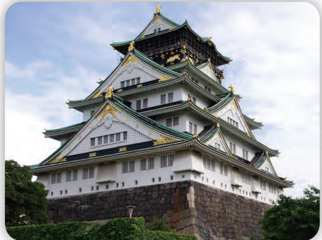
Shikkui on exterior and interior walls of Osaka castle, Japan
