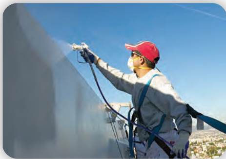
Machine application using Graco airless sprayer
