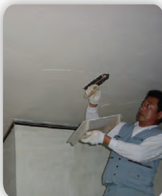
Hand application of Shikkui onto ceiling
